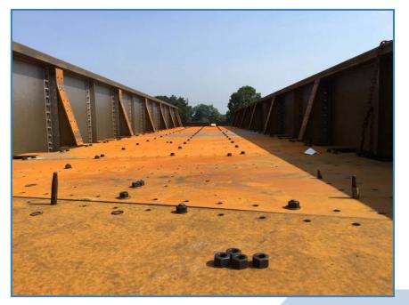
Steel pre-assembled in Fabricator's yard, disassembled, then trucked to site
